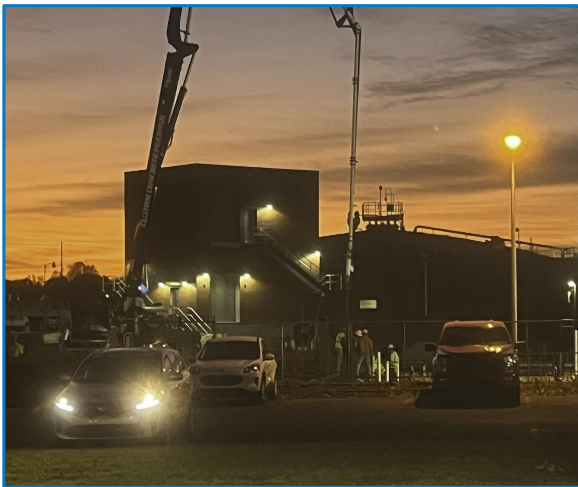
Energy Recovery Improvements Project - Concrete Pour at Dawn
