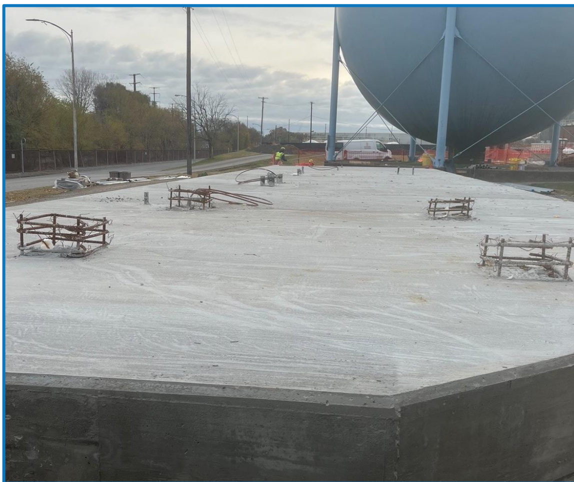
Finished 62-foot Concrete Foundation for the New Gas Purification Equipment
