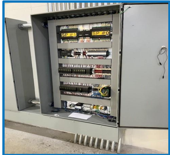
Refurbished PLC control panel 16/16A.
