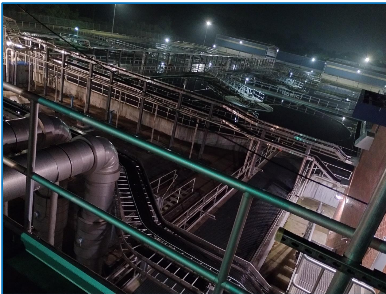
Nighttime view of the Final Clarifiers from the RAS Regeneration Tank. Photo by David Toth.
