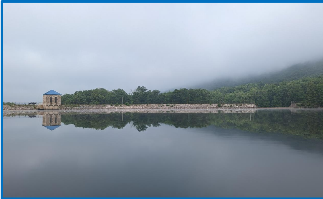
Intake Tower and DeHart Dam Breast
