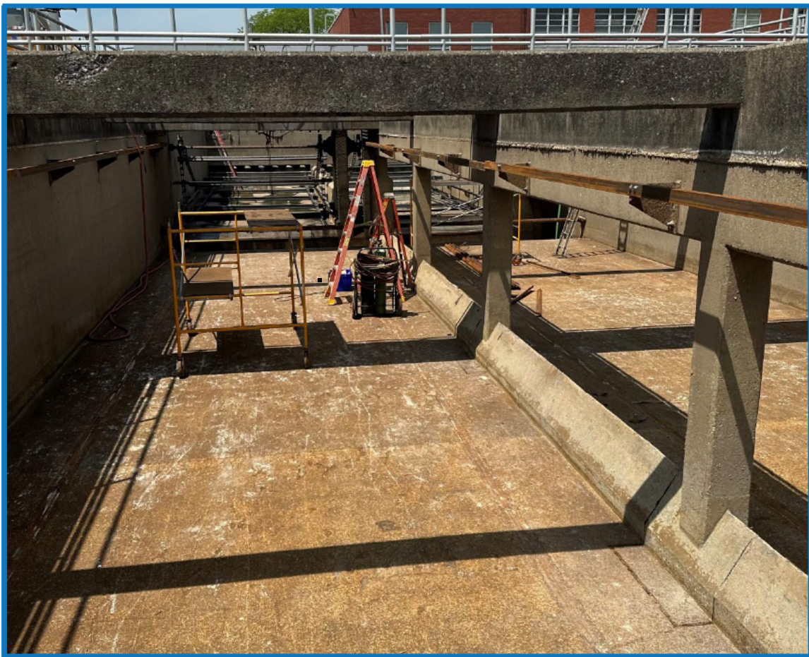
Rail fabrication for Primary Clarifier No. 4 continues
