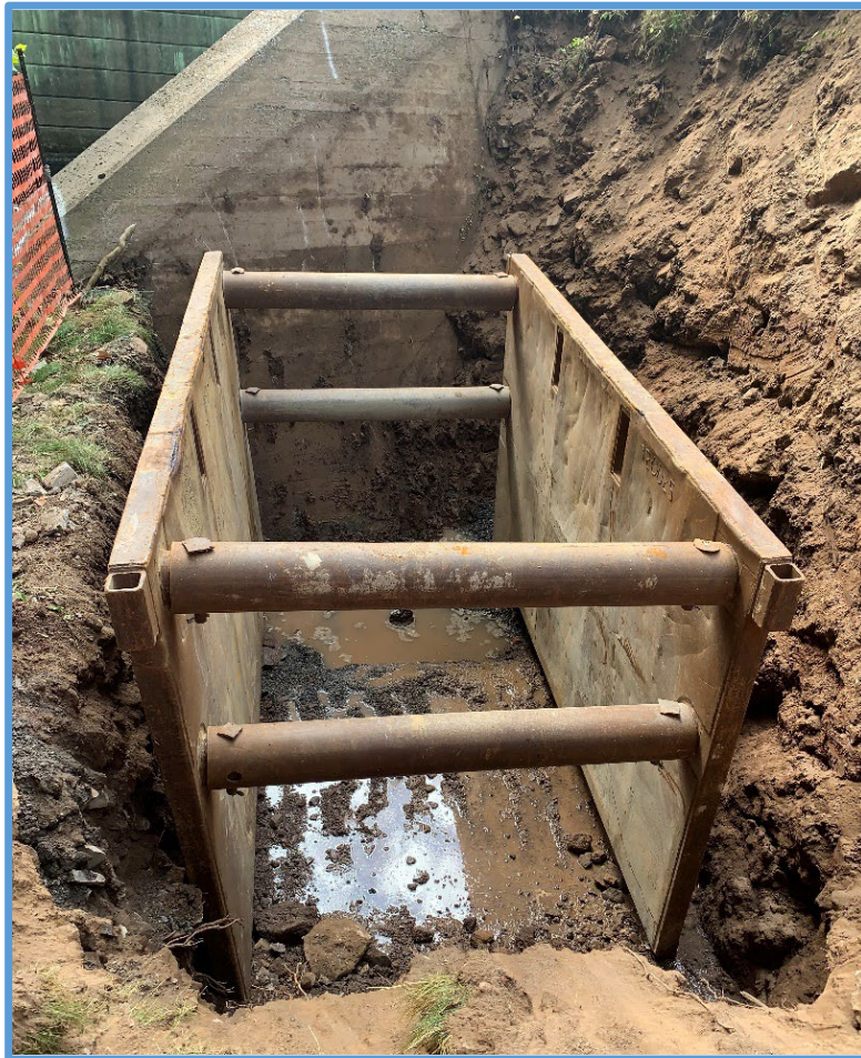
Transmission main excavation at Stoney Creek.
