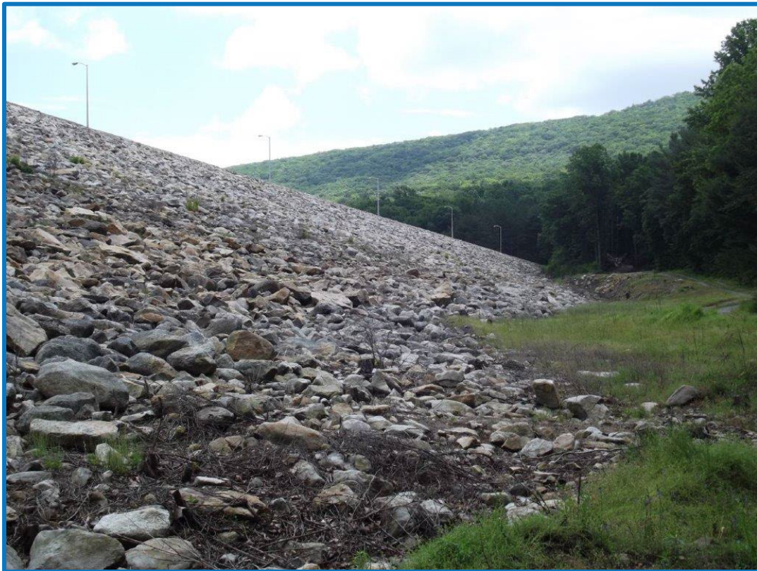
DeHart Dam Breast Looking South
