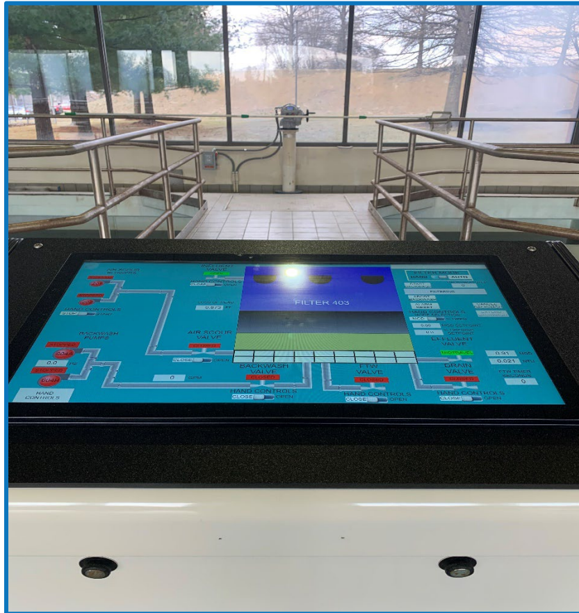
Ongoing filter console upgrades.
