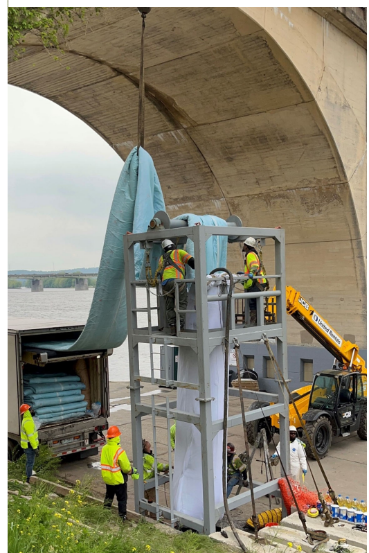
Figure 3.2-2: Front Street Interceptor Rehabilitation
