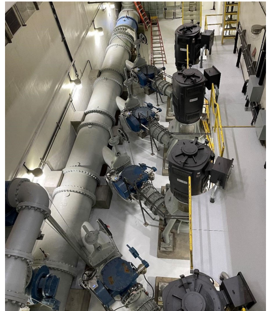
Figure 3.2-1: Front Street Pump Station Rehabilitation
