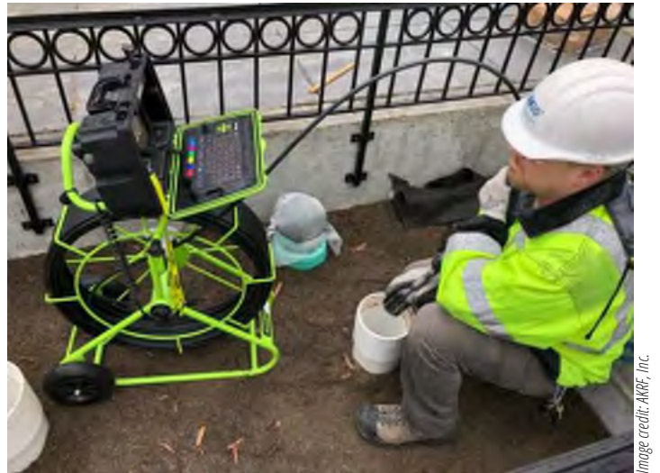
Inspector using a CCTV camera to observe pipes.
