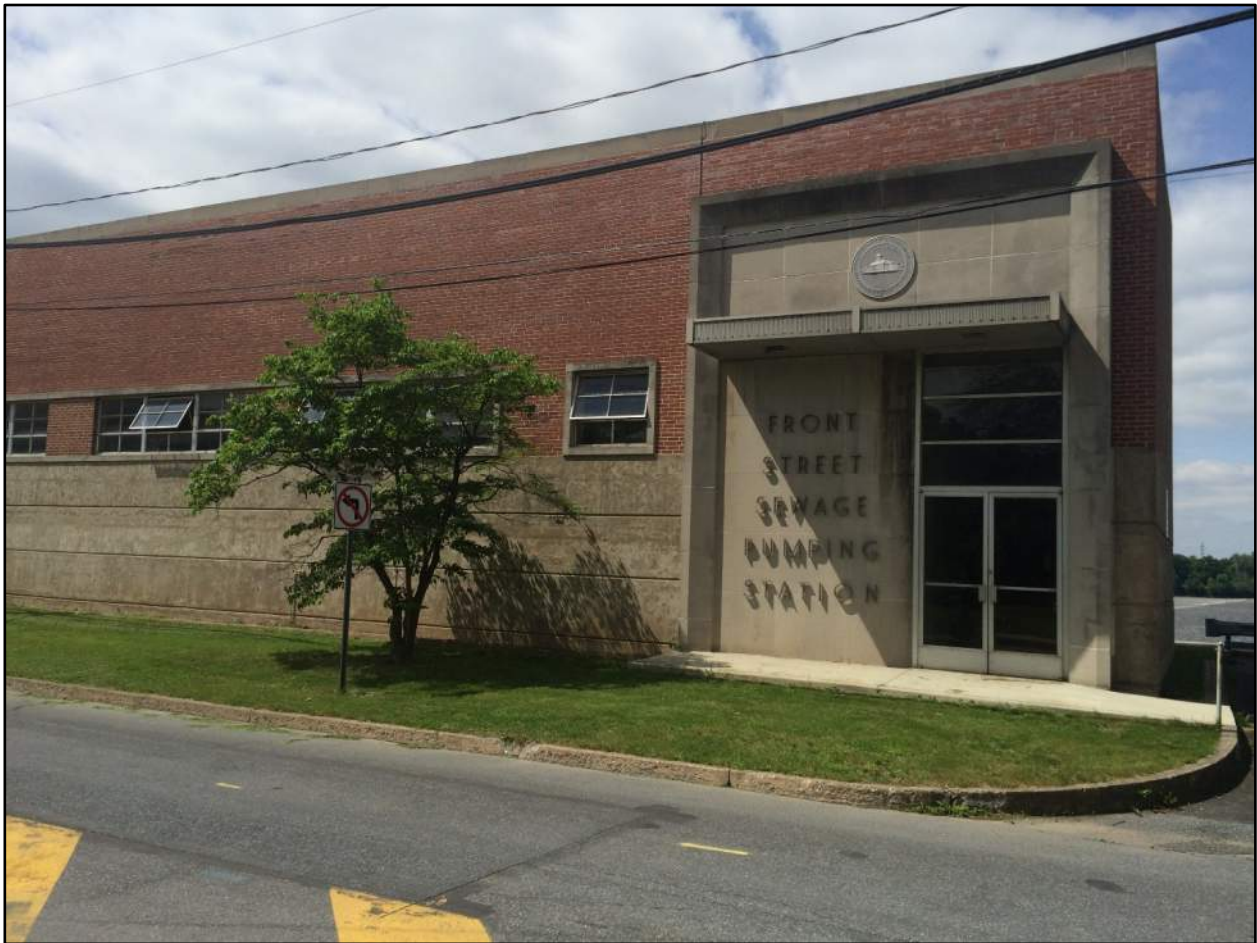
Figure 4.3-1 Front Street Pump Station
