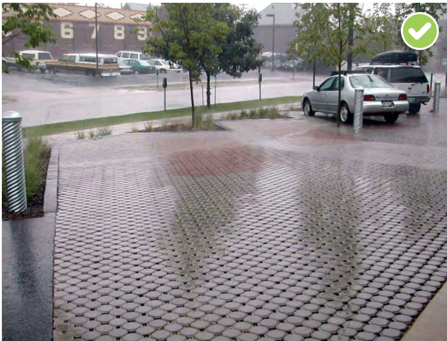
Clear surface and joints contribute to well-draining and functioning interlocking pavers.
