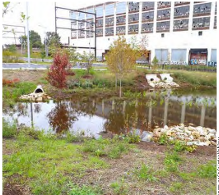
A well-kept stormwater basin.
