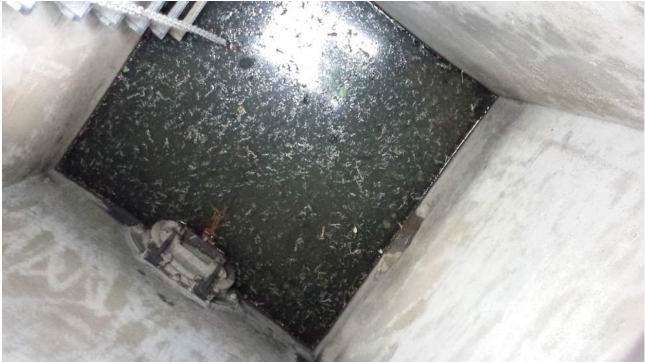
Flood Chamber with Flood Gate shown
