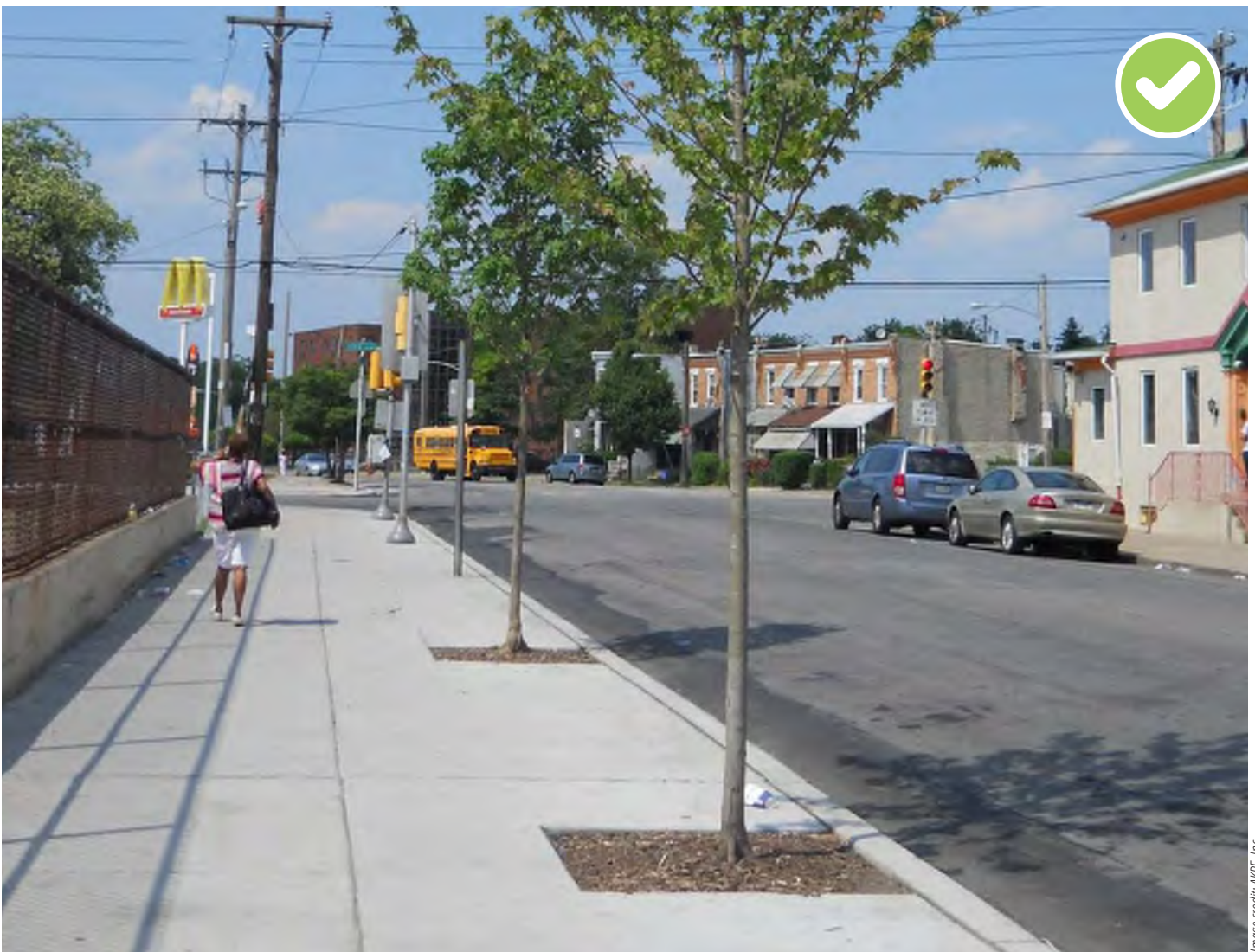
Healthy trees and sidewalks swept clean from trash and debris represent a well-maintained stormwater tree trench.
