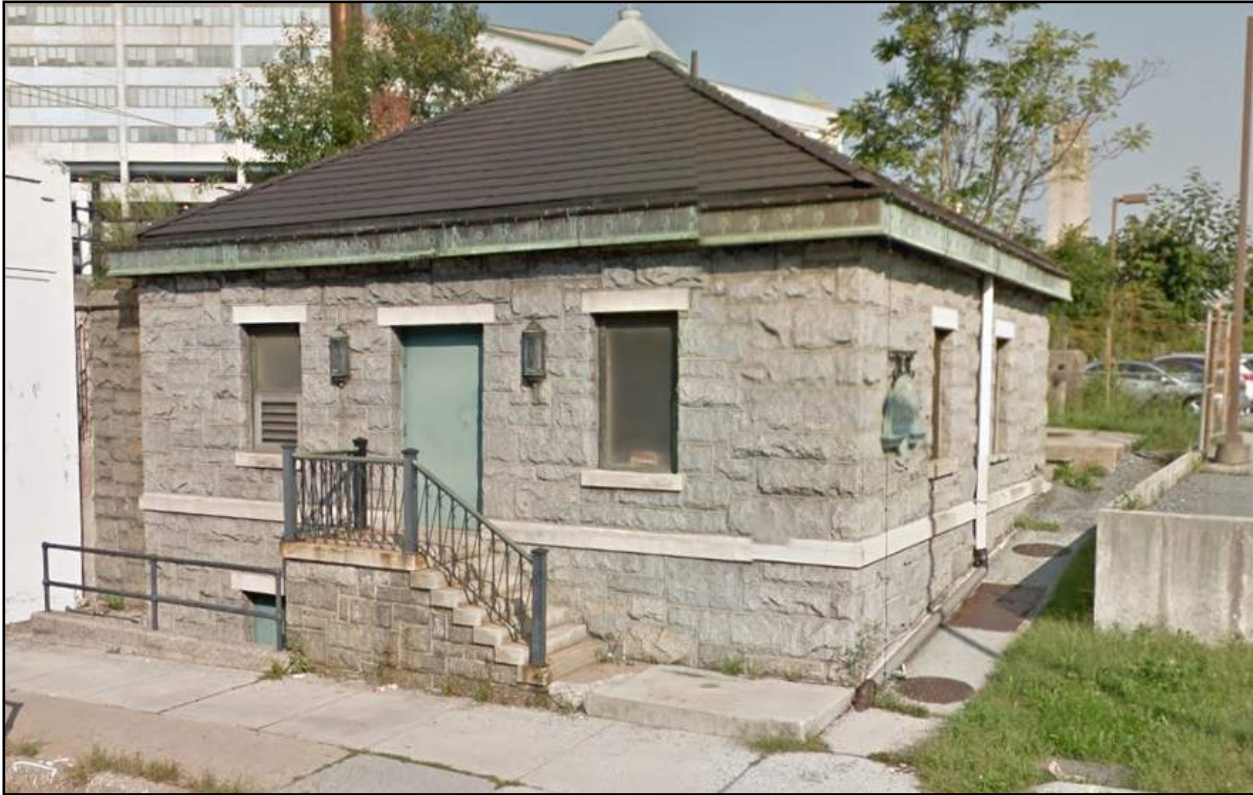
Figure 4.3-13. Market Street Pump Station
