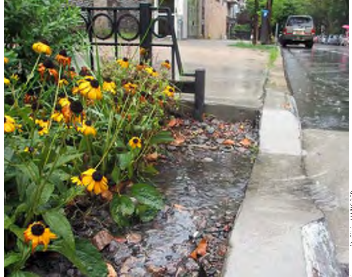
A clean and clear curb cut allows stormwater runoff to easily flow into the stormwater planter.
