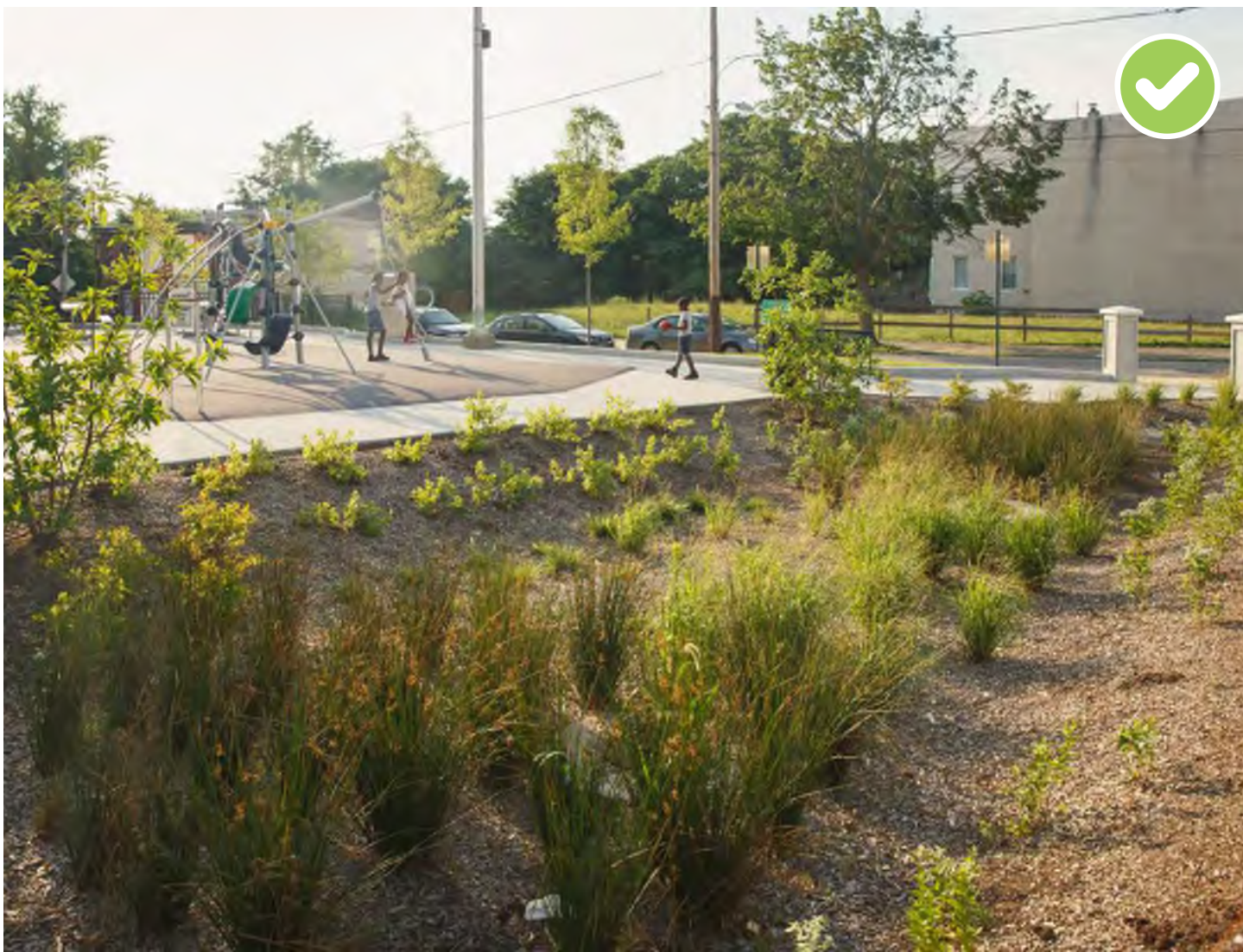
This newly planted rain garden built in at a playground manages runoff from the site and surrounding roadways.
