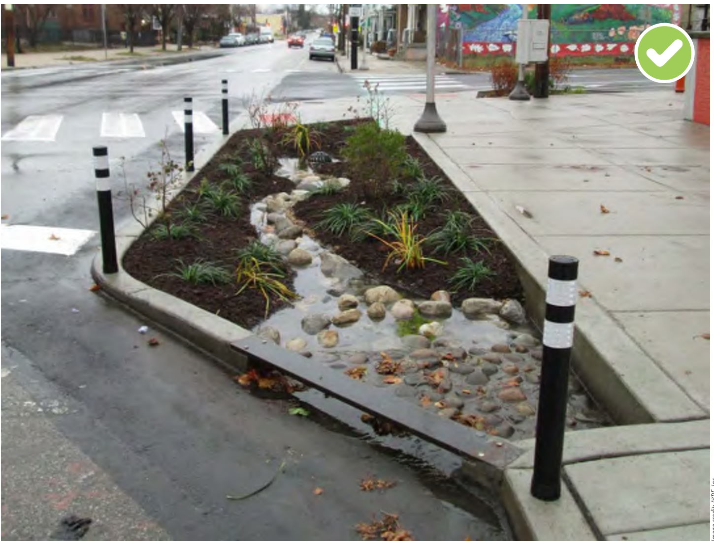
This stormwater bumpout exemplifies a well-maintained and highly functional feature.
