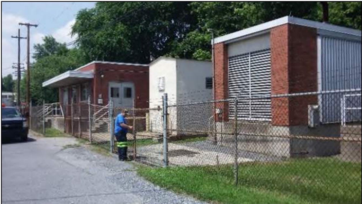
Figure 4.3-7 Spring Creek Pump Station
