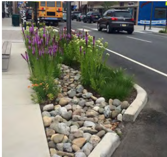
A stormwater bumpout with a clean and clear inflow point and thriving vegetation.
