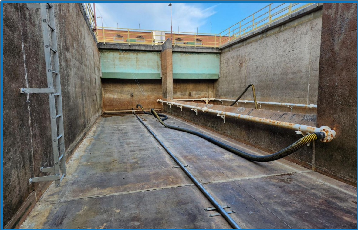
Basin Cleaning at Water Services Center
