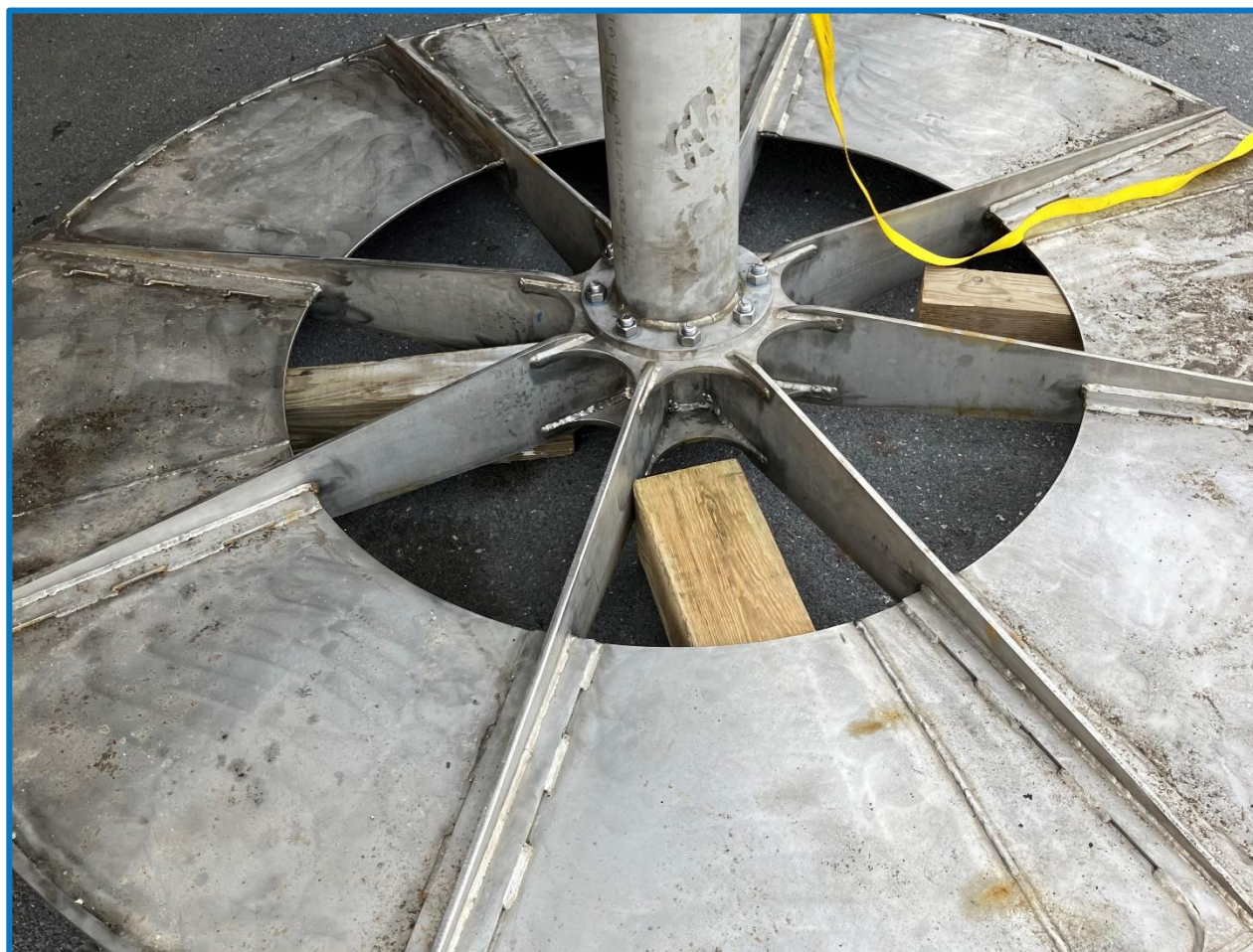
New Linear Motion Mixer Blade for installation on Primary Digester No. 2.
