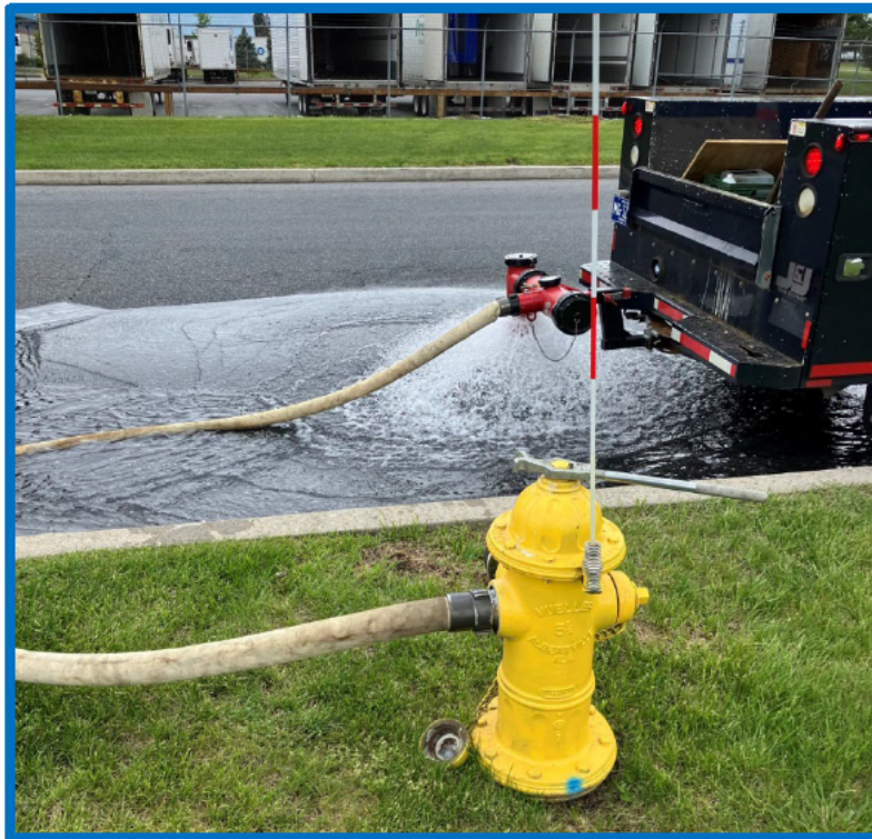
2023 Hydrant Flushing
