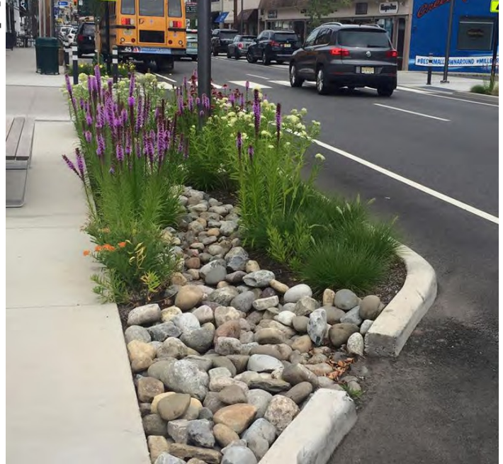
A stormwater bumpout with a clean and clear inflow point and thriving vegetation.
