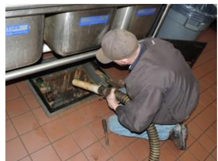
Figure 3: Clean grease traps a minimum of once per week. Increase the frequency if the total volume of grease and solid material displaces more than 25 percent of the total volume of the unit.
