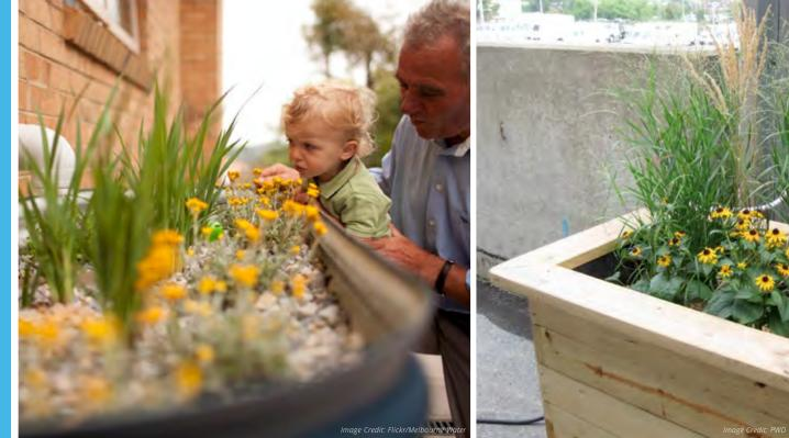
A flow-through planter is a box with soil and plants that sits on the ground, typically located next to a building. The stormwater from the building's roof is directed to the stormwater planter through a downspout. Stormwater filters through the soil in the box.
