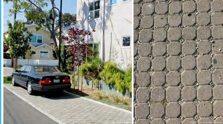
Pervious, or porous/permeable, paving is a special type of paving that allows stormwater to pass through it instead of running off of it. Pervious paving can be used in many places where traditional paving is used, particularly areas that do not have a lot of traffic, such as walkways and parking areas. An underground storage system usually sits below the pavement to store the stormwater.
