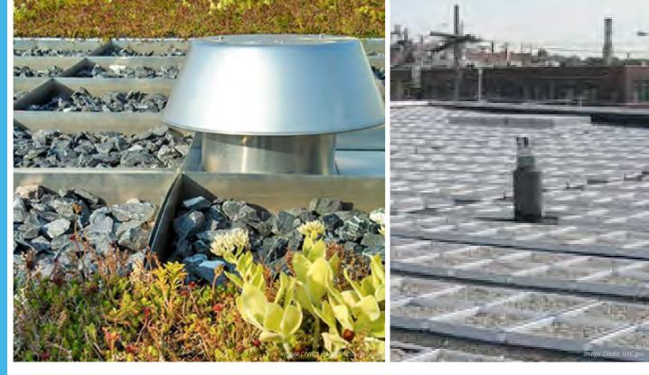
A blue roof is a roof that is either partially or fully covered by a system of stone storage trays. The storage trays capture rainwater until it evaporates. Blue roofs vary in size and can be used alongside green roofs.
