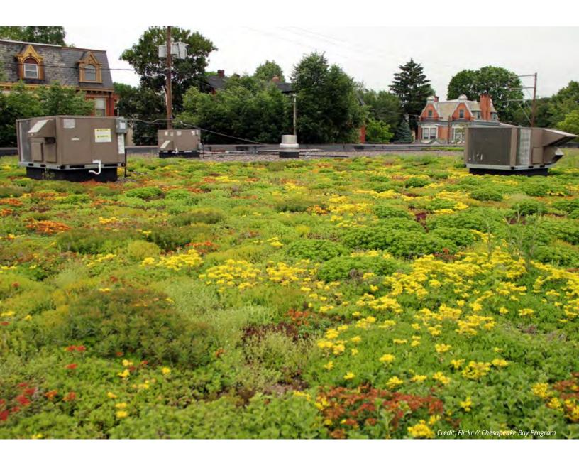
Higher maintenance is required until roof vegetation is established. Regular maintenance includes clearing debris, working to avoid plant loss, and checking for damage from environmental conditions. Ensuring that installed plants, growth medium, and other drainage materials are tailored to the specific environment (climate, building surroundings, etc.) can reduce maintenance requirements.
