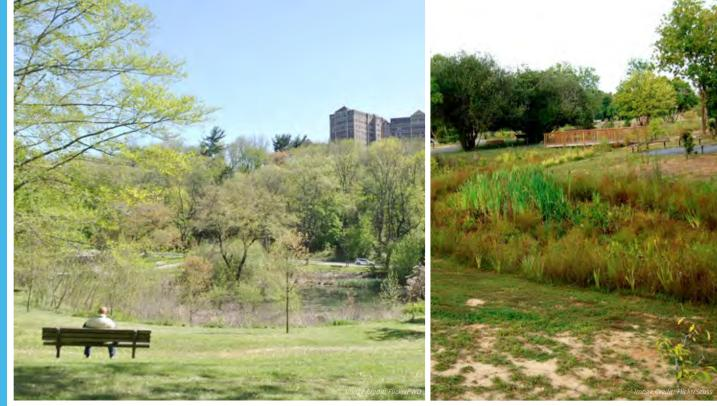
A stormwater wetland is a constructed area with soil, plants, and marshy water. Stormwater wetlands typically include a small pool that filters some pollutants out of the stormwater and then a larger area of with marshland vegetation that treats and filters the water similar to a natural wetland. Stormwater wetlands can serve as habitat for wildlife.
