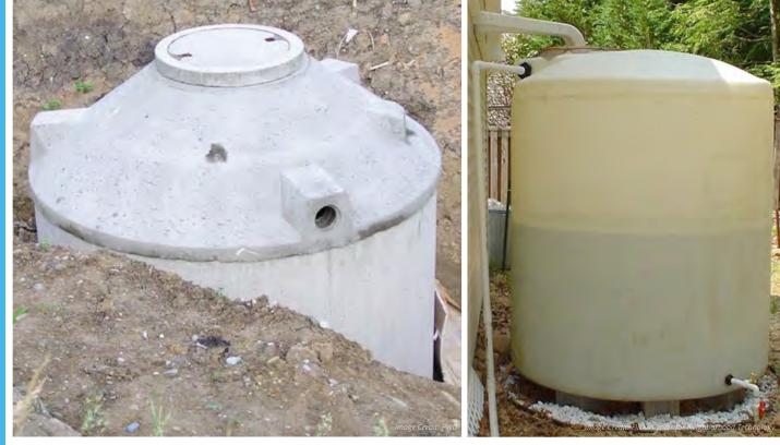
Cisterns are large, enclosed structures that can sit on the ground or be buried below ground. Stormwater is directed to cisterns through downspouts or pipes. Stormwater is stored in the cistern until it is needed for another use. The collected water is often used for things that do not require drinking water, like watering plants or washing cars.
