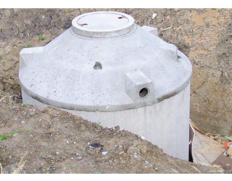
at a controlled rate to ensure that there is available storage for subsequent storm events. Depending on the stormwater objectives or goals of a site, cisterns may need to be used in conjunction with another practice.
