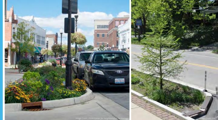
A stormwater bumpout is an area with soil and plants that extends out from the existing curb into the street, with a new curb at the street edge. They can be put at the corner of a block, in the middle of a block, or along the entire length of a block. The soil and plants are lower than street level to capture stormwater from roads and sidewalks. Stormwater bumpouts can vary in size and materials.
