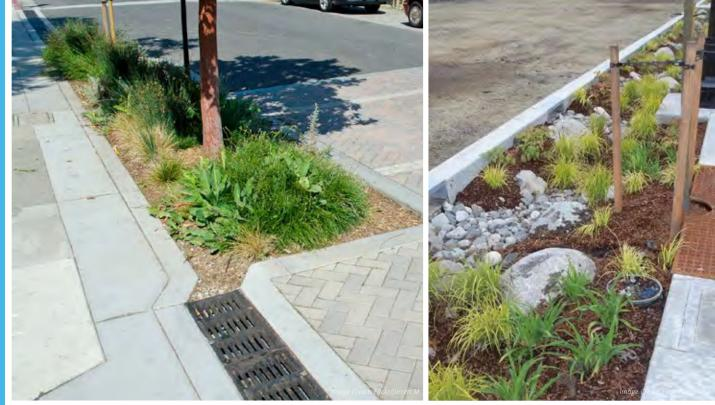
Green gutters are continuous, narrow areas with soil and plants that are put along the edge of a street where it meets a sidewalk, with a new curb at the street edge. The soil and plants are lower than street level to capture stormwater from roads and sidewalks. Green gutters can vary in size and materials.
