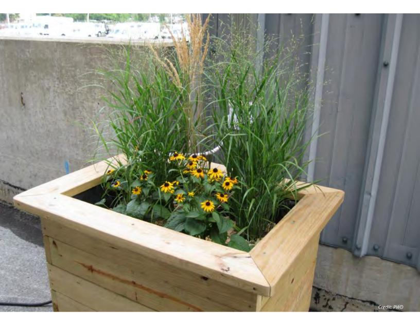
Depending on the size of the planters and the materials used, flow-through planters are a relatively inexpensive way to manage stormwater. However, the amount of stormwater a flow-through planter can manage is limited to runoff from the adjacent structure's roof. Maintenance of the planter itself is minimal once vegetation is established. As with many other types of GSI, careful consideration should be given to selecting native, or adaptive, water-tolerant plantings.
