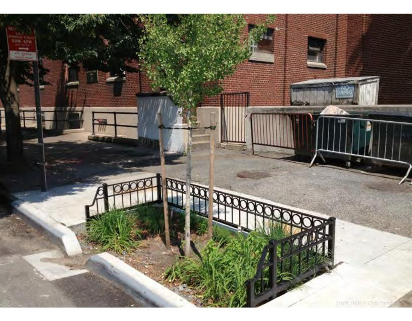
Stormwater trees increase tree canopy and increase air quality while enhancing streetscape. However, unlike a typical street tree, stormwater trees need to be able to handle larger volumes of water entering through tree pits. Therefore careful selection of native, or adaptive, water-tolerant trees is necessary to ensure tree health. Maintenance requirements include trimming limbs, removing debris, and occasional evaluation to ensure that the trees remain healthy.
