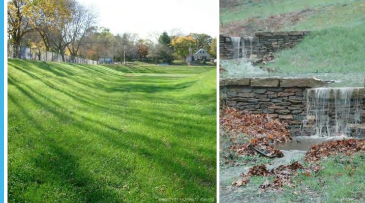
A stormwater basin (detention/retention pond) is a sunken, usually grassy area that is designed to collect and store stormwater. Stormwater basins vary in size and can either slow the stormwater until it is treated elsewhere, or allow it to drain into the soil. Vegetation improves filtering, water quality, and the aesthetics of the basin.
