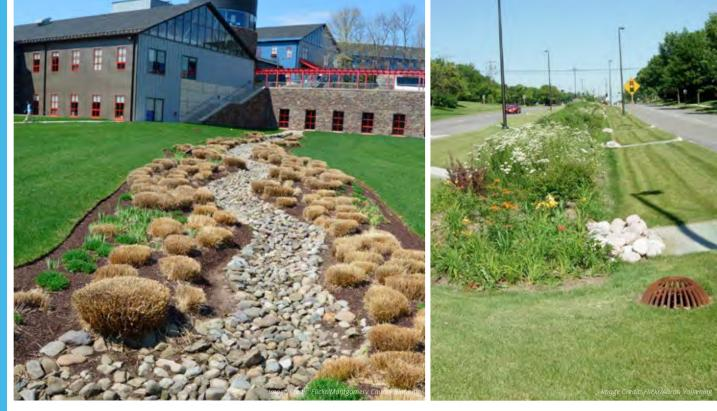
A bioswale is a long, shallow depression designed to slow the flow of stormwater and allow it to drain into the soil. Swales can be used as an alternative to traditional ditches or as a way to slow stormwater before it gets to other GSI.
