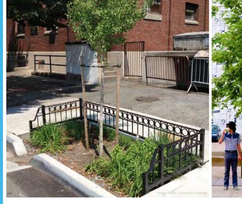
A stormwater tree is a street tree planted within soil that is lower than street level to capture stormwater from roads and sidewalks. The tree absorbs stormwater through its roots. Some stormwater tree pits have metal grates above them. Others have inlets that direct stormwater to the trees.
