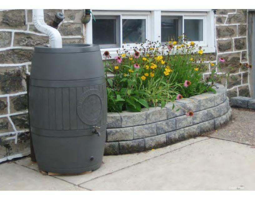
Most rain barrels are prefabricated which reduces the overall cost and maintenance requirements. However, due to their small size, the potential stormwater benefit is limited. Aside from ensuring roof leaders are clear of debris and regularly using the stored water, maintenance of the system is minimal. Rain barrels should be completely enclosed or have appropriate screens to control mosquitoes and should be completely emptied when temperatures fall below freezing.
