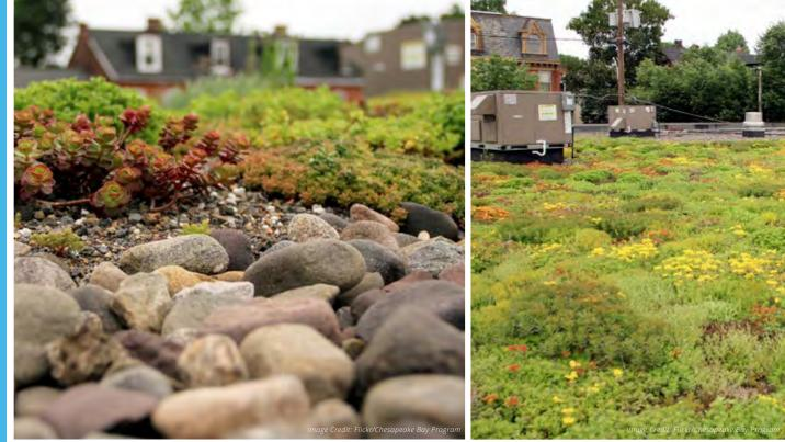
A green roof (or vegetated roof) is a roof that is either partially or fully covered by a system of plants. The plants are put on top of soil or a water storage system. Green roofs vary in size and depth depending on the weight the existing roof can handle.
