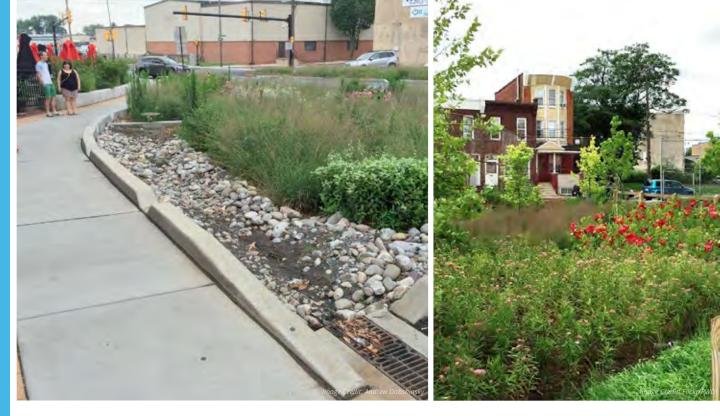
A rain garden is an area with soil and plants that is not surrounded by a curb. Rain gardens are typically located in grassy areas. The soil and plants are lower than surrounding areas to capture stormwater. The stormwater collects in the rain garden, creating a small, shallow pond until the water drains down through the soil. Some rain gardens have an underground storage system beneath them to hold more stormwater. Rain gardens can vary in size and materials.
