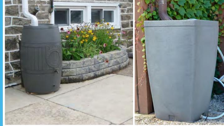
Rain barrels are enclosed, typically plastic or metal structures that sit on the ground, typically located next to a building. The stormwater from the building's roof is directed to the rain barrel through a downspout. Stormwater is stored in the rain barrel until it is needed for another use. The collected water is often used for things that do not require drinking water, like watering plants or washing cars.
